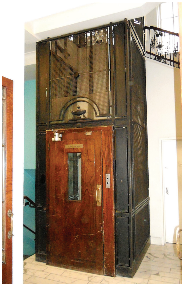
Painted décor at back of shaft, which was very dark, much improves the appearance of the ground floor entrance.
