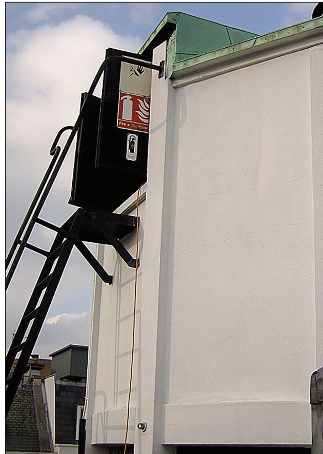
Machine Room Access.
