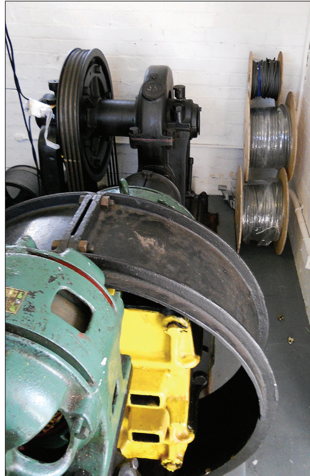
New ropes stored in motor room, ready for installation.
