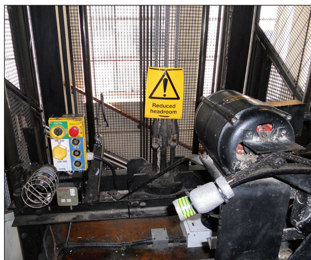
Repositioned top of car inspection box.
