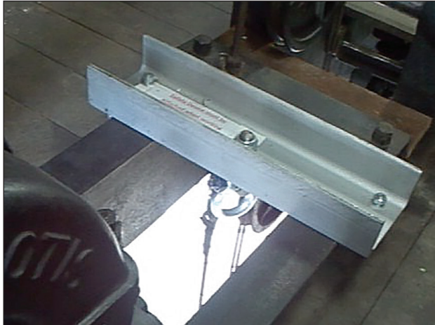
The hook on the sling can be connected to an eyebolt fixed to parallel flange channel across the machine support channels.
