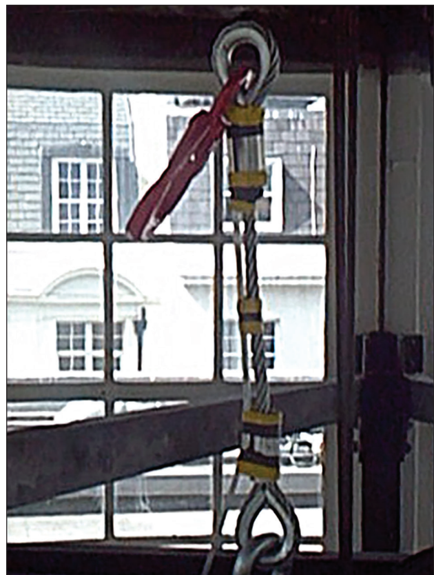
Sling on the frame of the Dome.
